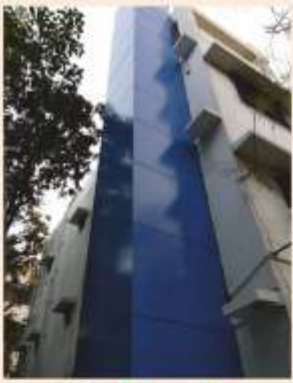
Lift Out side covering
